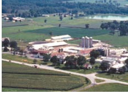
Aerial view of the Dairy Research Facility and surrounding area on the east side of BARC, circa 1994.
